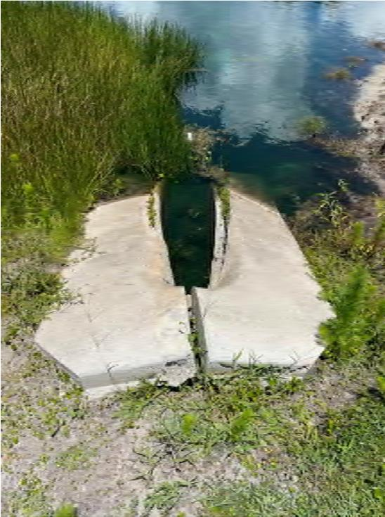
**Location 13:** Remove and replace mitered end section top. Add bahia sod around structure, with 57 stone and compacted fill beneath concrete to ensure level placement and prevent undermining/erosion.
