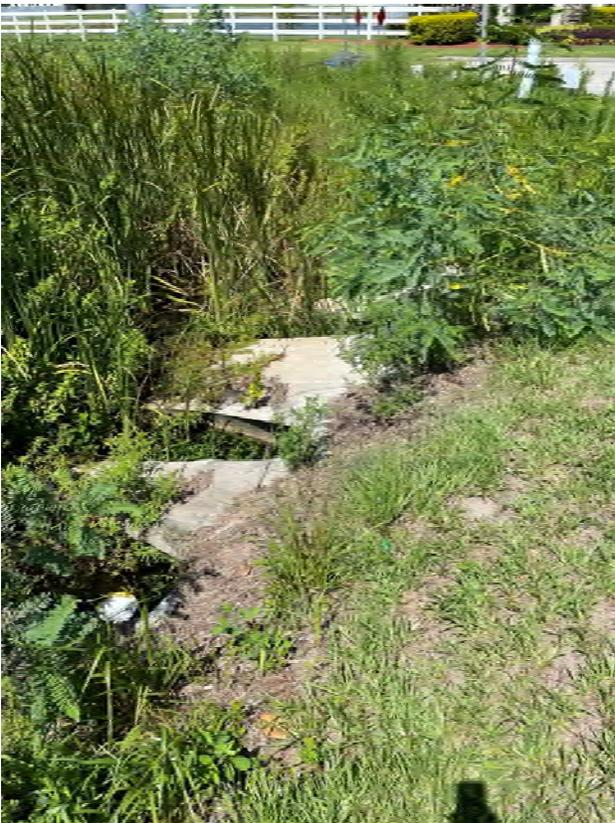
**Location 4:** Remove vegetation/sediment inside and within a 6' radius around end treatment, to provide positive discharge of stormwater.
