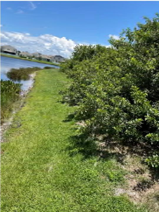
**Location 20:** Invasive vegetation growing onto pond berm. Remove approximately 5'x250' of vegetation to prevent turf deterioration/erosion.
