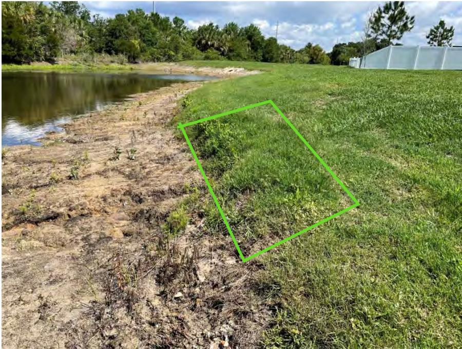
**Location 2:** 5'x5' section of pond bank is eroding underneath the sod. Restore pond bank according to attached pond bank repair detail.
