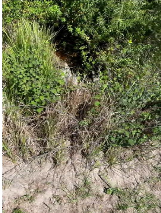
**Location 7:** Clear 6' access path and remove sediment/vegetation within 6' radius around end treatment to provide positive discharge of stormwater.
