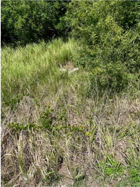
**Location 5:** Clear 6' access path and remove sediment/vegetation within 6' radius around end treatment to provide positive discharge of stormwater.
